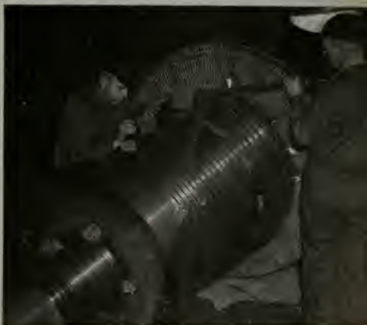
At bottom, left: Installing labyrinth packing in backing turbine diaphragm. Right: Installing blading segments in LP rotor
